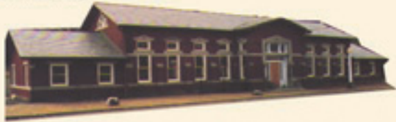
Built in 1880 for the P.C. & O. R.R. and nicknamed the "Pan Handle Depot", this historic railroad station, more accurately referred to as "Pennsylvania Station" serves as offices for The Evans Foundation as well as other community service organizations. N23-O
